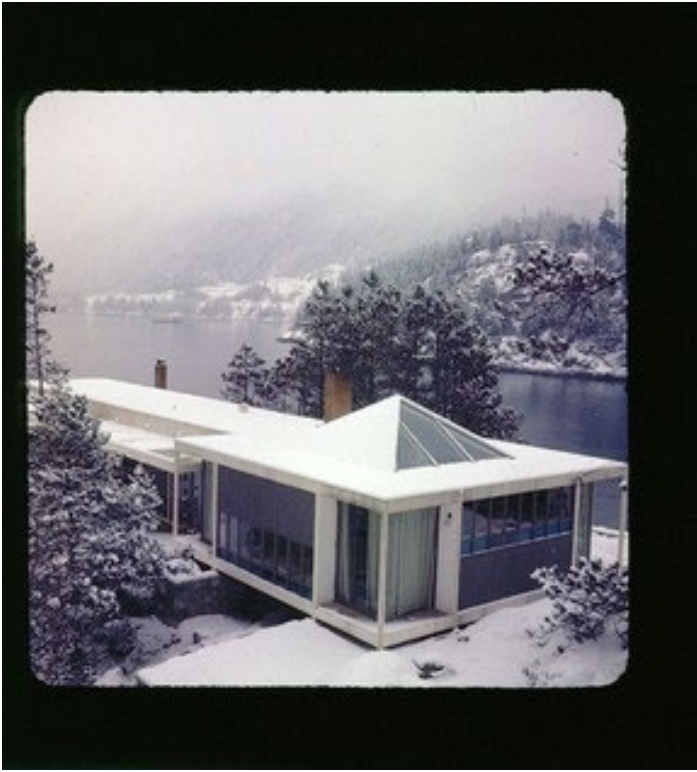
Massey residence, 1955, Arthur Erickson and Geoffrey Massey architects. Vancouver Sun
